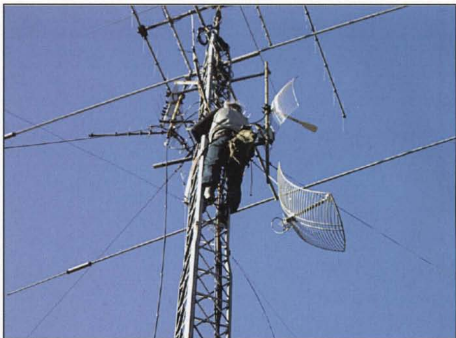
Photo D. This is Robert "Bob" Morgan, WB5AOH, mounting HSMM antennas on the Austin Texas Red Cross Tower, which is part of the AARC club station, W5KA. (Photo credit David, AD500)
