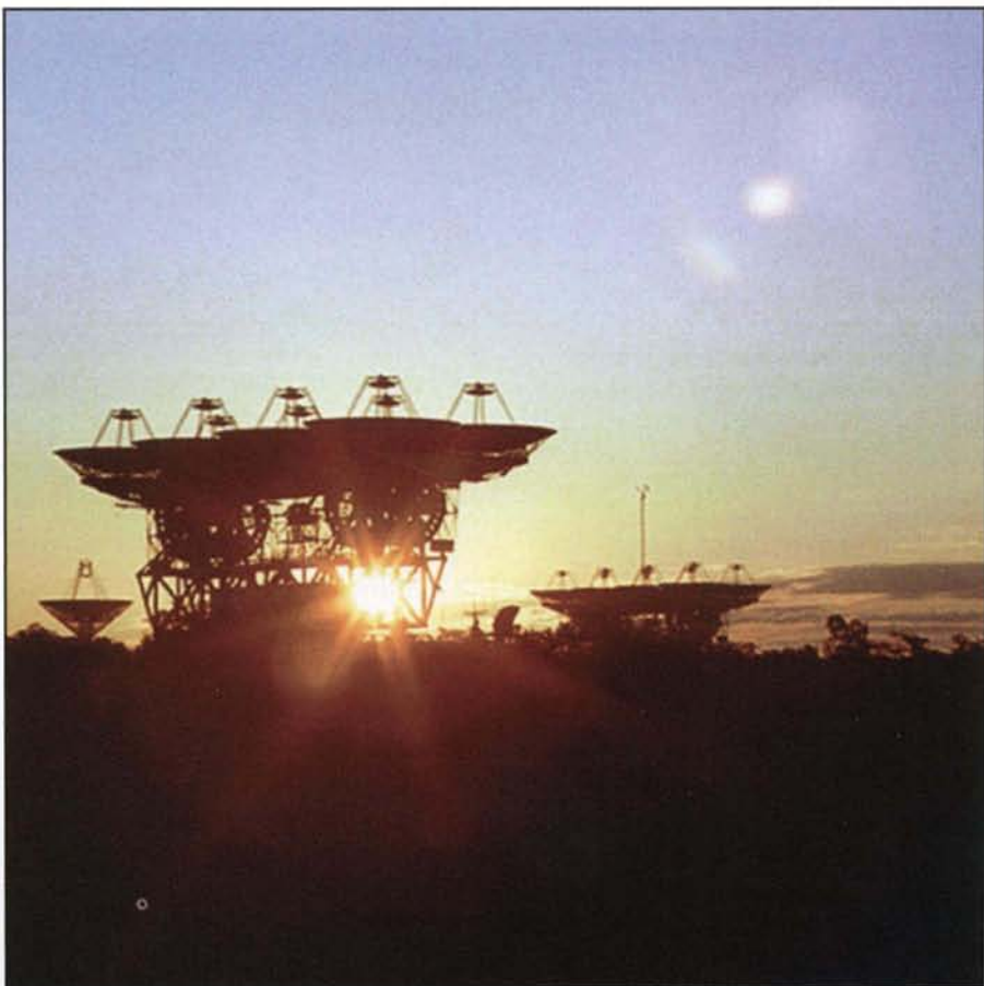
Figure 1. On November 19, 1962, three scientists from the Russian Institute of Radio Engineering and Electronics succeeded in bouncing the word "Mir" in slow-speed Morse code off the surface of Venus and received their own echoes. They used the 50-kW transmitter of the Evpatoria Planetary Radar in Crimea, Ukraine, into an array of eight 16-meter parabolic dishes.
