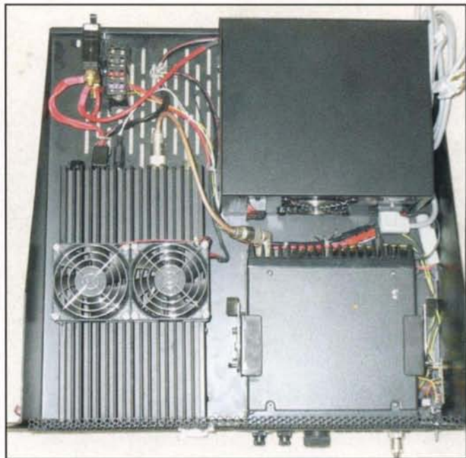
Photo 4. The beacon equipment layout.
