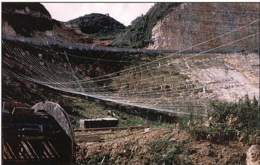
Photo C. Contrary to the patent filed by the General Bronze Corporation, the final design of the Arcibo dish used steel cables draped across the valley and used to support a wire mesh surface.
