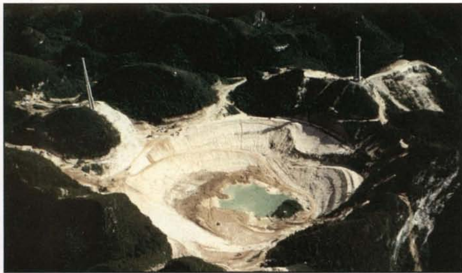
Photo D. The dish feed was also suspended by steel cables, but from three great towers as shown in this photo from 1961.
