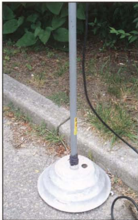
Photo F. This is a view of the umbrella stand with concrete added and the first mast section installed. A piece of cloth held by electrical tape is wrapped around the connecting area between the stand and the mast in order to stop movement during windy conditions. This base is not quite flat and so a wrench was placed underneath one side for more stability. Caution must always be exercised when considering how high an antenna can be placed. If it is windy, it is best to keep the height to 15 or 10 feet.
