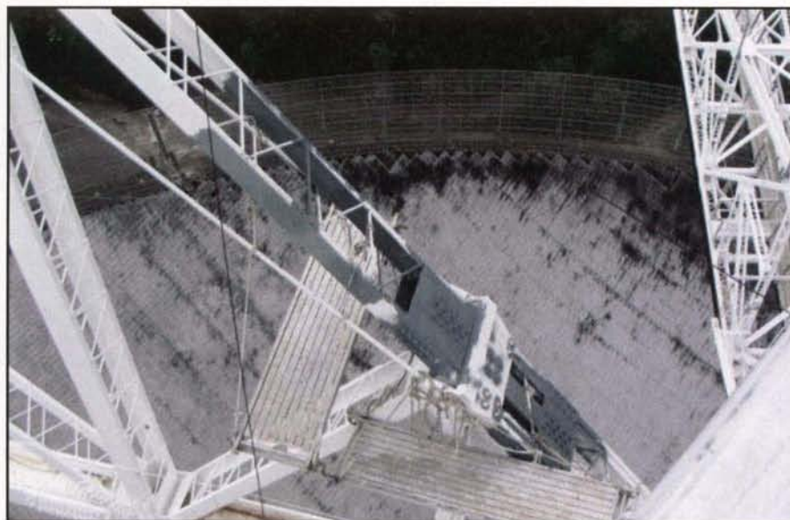
Structural repair site, with the main dish surface 450 feet below.
