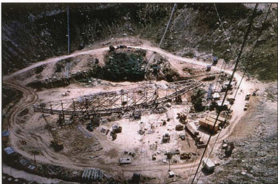
Photo E. The massive size of the feed assembly of the Arecibo dish.
