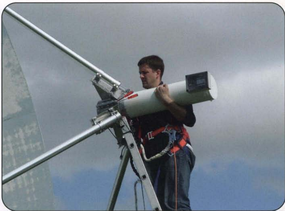
Christoph Joos, HB9HAL/HB9MOON, installing the OM6AA designed dual-mode, septum polarizer at HB9MOON's 10-meter EME station. (Photo courtesy of HB9HAL)
