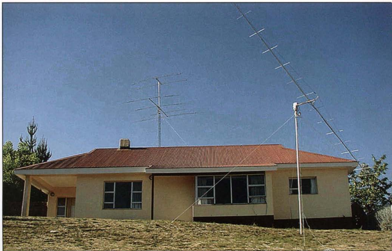
Photo F. 7P8/ZS5JR, one Yagi with azimuth and elevation rotor.
