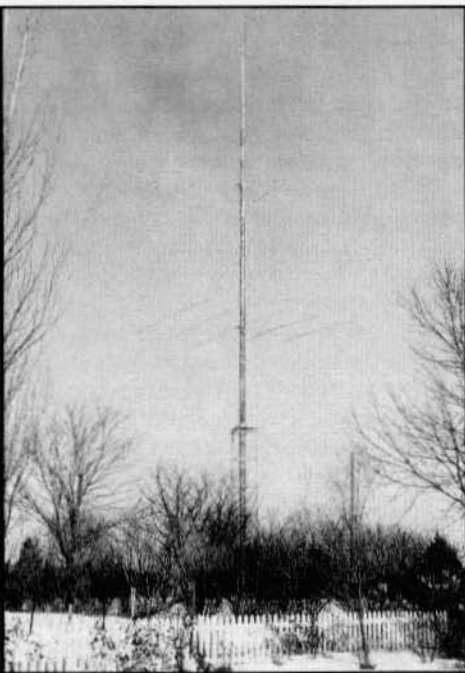
Lee installed yagi's for 10 and 20 meters on the tower in 1951
