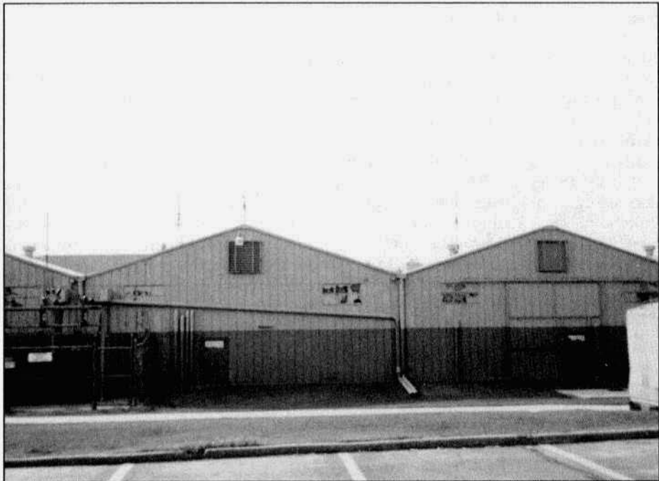
The famous 'Butler Building' where most of the Collins SSB gear was developed.
