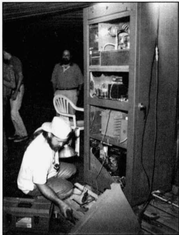
Tim Smith, WA1HLR, repairing the plate transformer on the homebrew transmitter.
