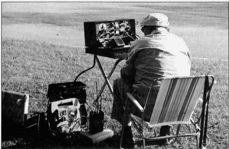
Phil Morse, W2WAX, on the air with a BC-474-A under field conditions—battery, inverter and AC supply—at Oxford Furnace Lane, New Jersey. Oxford Furnace is where George Washington's cannon balls were cast for the revolutionary war.
