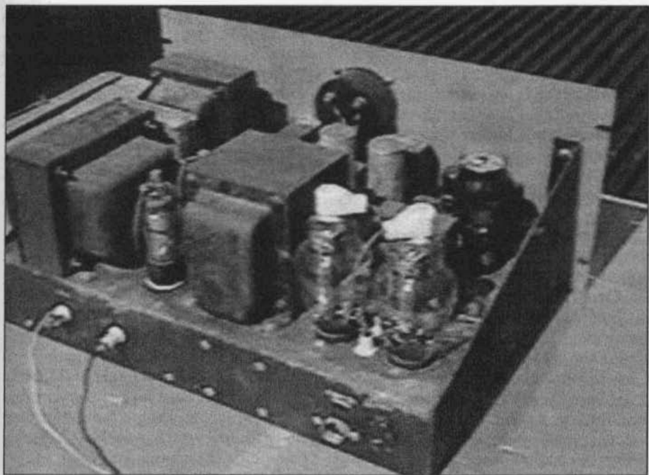
The modulator deck before restoration
