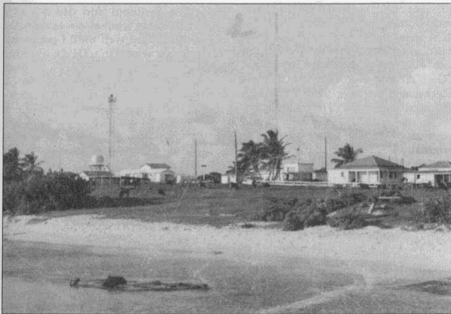
A view of the Swan Island facility from the dock area.
