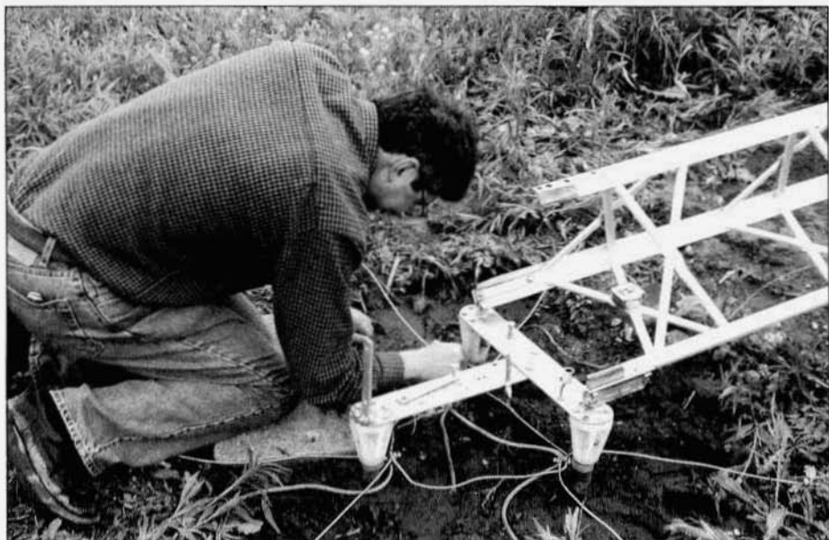
Phil Sanders wires the ground field at the base of the Hy-tower. As a new ham first licensed in the spring of 1999 and upgrading to Extra by the end of the year, Phil found this experience is 'A real kick'.
