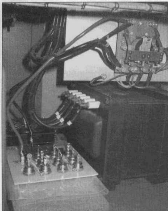
Figure 5. Limiter temporarily installed in KW-1.
