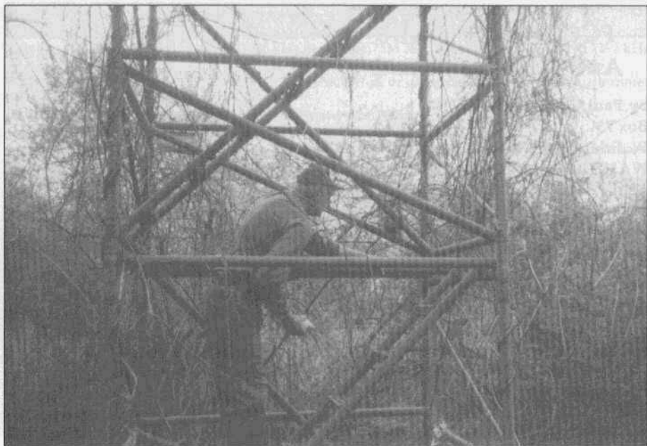
This is an ex-military airport control tower recently acquired by George Rancourt, K1ANX. The 48' tower is 6'x4' at the base and is comprised of 6 foot sections with stairs between sections. The guys are all stainless steel.
