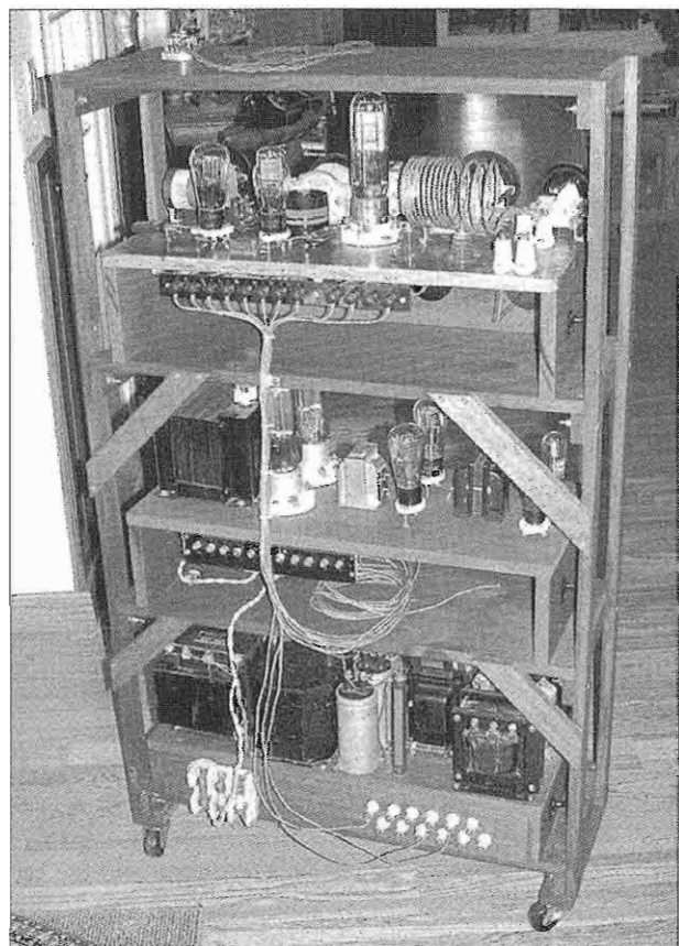
Martha's backside during construction of the interconnect wiring harness.
