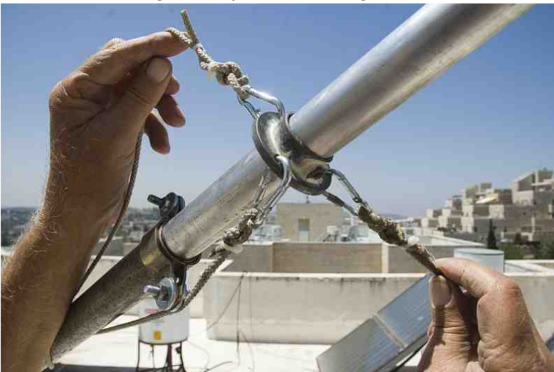
Pic 3: The omega clamps and a flange at 4X4LH's roof
