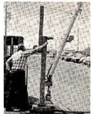
Tilting the tower over is a one-man task with the Wilson bases.
