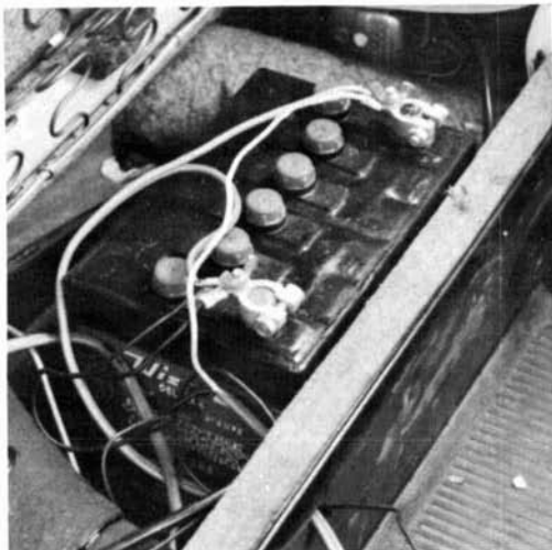
Heavy-duty battery under the rear seat is used exclusively for the radio gear (can also be used for starting the car on cold winter mornings).
