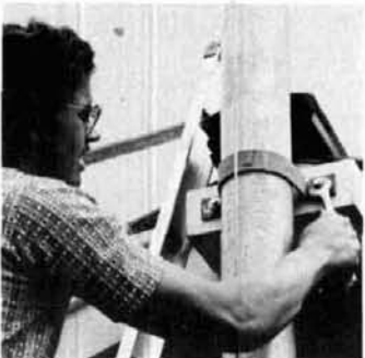
Mounting the House Bracket
