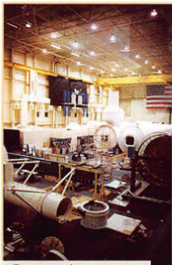
Construction de la station ALPHA.
