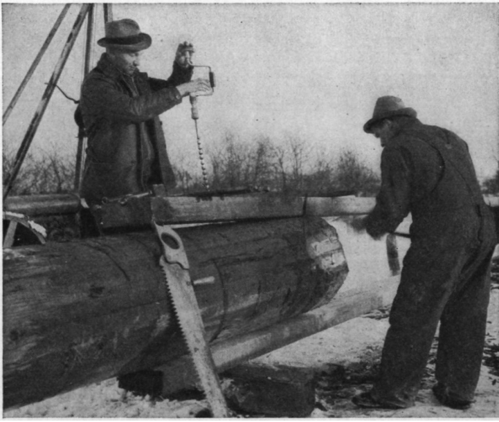
FIG. 3.112. The beginning of a pole-splicing operation and the construction of a butt-spliced pole. (Photograph courtesy of National Broadcasting Company.)
