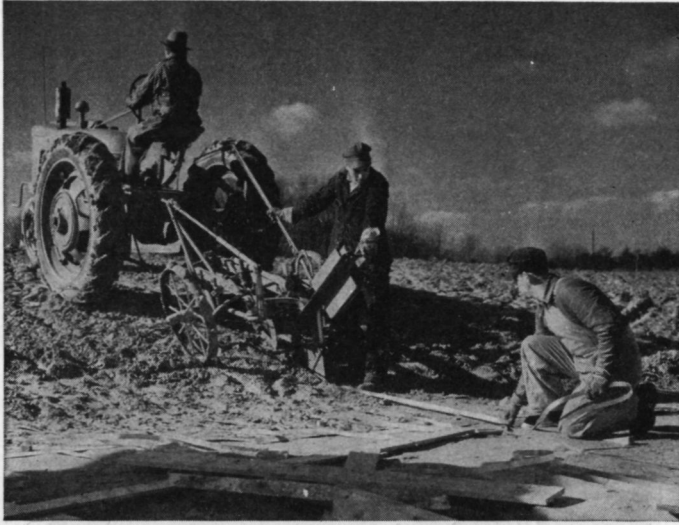
FIG. 2.67. A tractor-drawn wire plow for burying ground wires. The plow blade is of sheet steel that cuts a thin furrow. The wire is fed into the furrow as the plow advances. Horse-drawn hand plows of similar principle are often used.
