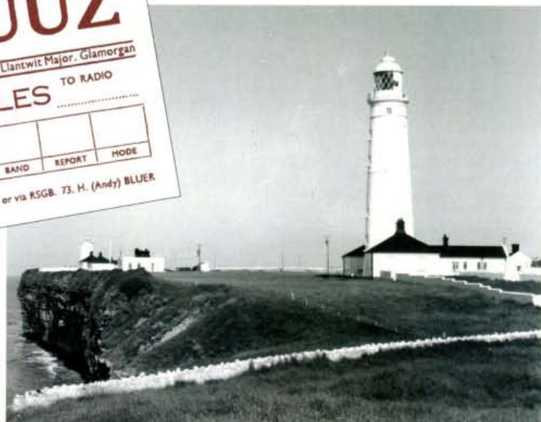
Fig. 2: Nash Point Lighthouse. Andy's second shack is the small building on the far right.
