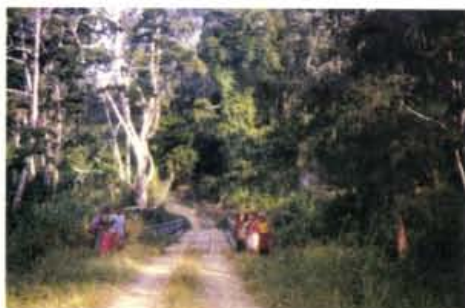
Fig. 1: Example of one of the better bridges in Gorokain.
