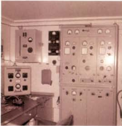
● Fig. 3: Radio station of MV Henri G/SLUR, 1959, showing main transmitters: 2MHz 'phone band (100W) m.w. (400W), s.w. 4-22MHz (400W), c.w. and voice.
