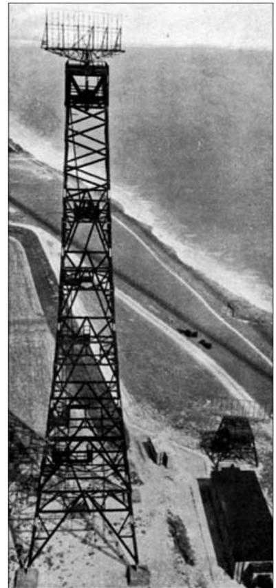
● A typical Chain Home Low (CHL) radar site, showing the 56m (185ft) steel tower with the rotating array mounted on top (see text).
