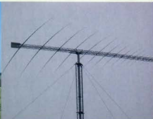
● Fig. 2: A Radio Amateur's dream antenna! A close-up view of the h.f. log periodic antenna. Formerly at the Post Office's h.f. site in North Weald in Kent, the antenna provide an extremely useful wide-band directional array.
