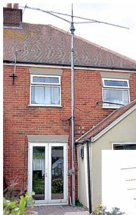
● Fig. 1: The author needed to take advantage of the reduced visual impact of a mast close to the house, but with little space or adequate supporting brickwork. Tennamast's solution was a 'gallows post', secured both to the wall and to a block of concrete beneath the patio...ideal for the 7.6/4.2m lightweight Adapt-a-Mast.
