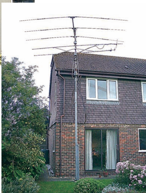
● Fig. 2: The Tennamast Standard tilt-over mast (10.7/6.4m) fits on a ground post. When retracted, the antennas are well below roof level, but can be raised well clear for operating. The ground post stands in a steel sleeve set in a cubic metre of concrete enabling the post to be easily removed...
