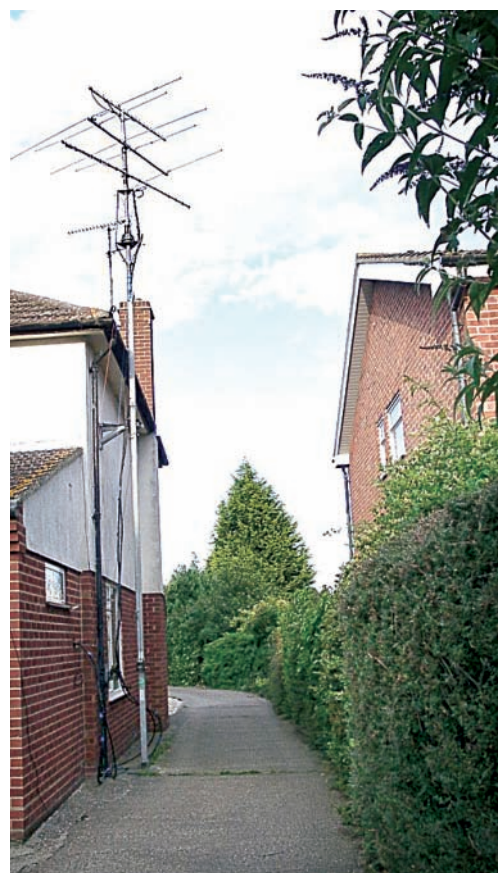
● Fig. 3: Extending to 12.2m (7.3m lowered), this Tennamast Standard Plus mast was originally attached by a strong bracket at bedroom-window level, tilting from the base (see text).
