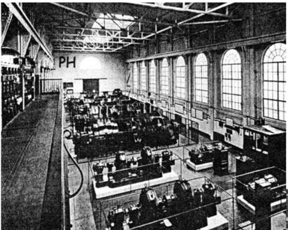
Fig. 2: A general view of the power plant. Three large sets at the rear were for GBR, each being capable of 500kW at 7kV d.c. A fourth large machine could supply 500kW at 12kV d.c. for GBY. In the foreground (left) are 2-200kW machines which generated (at 100Hz) the filament supplies for GBR and GBY and (right) smaller sets that provided lower voltage auxiliary supplies.
