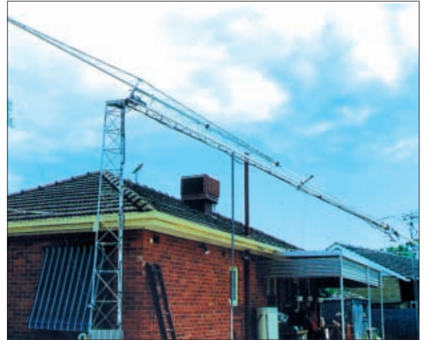
● Fig. 1: The mast on the 'folded' position, that allows work to be carried out on an antenna single handed.
