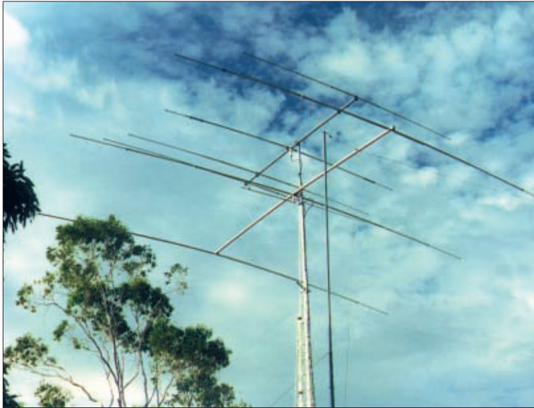
● Fig. 1: The mast on the 'folded' position, that allows work to be carried out on an antenna single handed.
