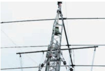
● Fig. 4: A cross-arm gives separate attachment point for long wire antennas, keeping them apart.
