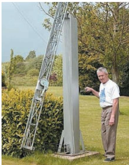
● Fig. 2: Waste not - want not! Utilising the top two sections of a failed Strumech tower on a home-made ground post. Roger is shown cranking up his 'little' mast.
