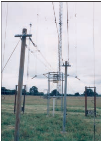
● Fig. 6: The photograph shows part of the antenna beam slewing system and although it may not be obvious...the pole and wires in the immediate foreground form a Pawsey stub familiar to Radio Amateurs! (See text).
