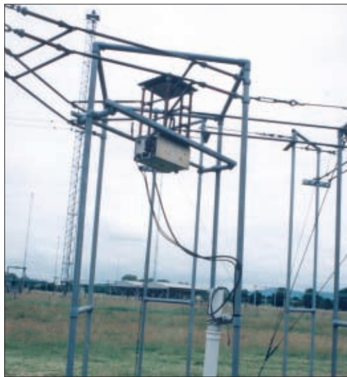
● Fig. 5: All antenna switching and transmission beam 'slewing' is carried out remotely with the aid of air operated switch gear. A slewing system for one of the main antennas is shown here (see text).
