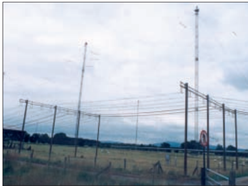
● Fig. 4: The antennas are fed by open wire feeders. Some feeders are of the familiar parallel wire type, although some sections (for matching and transformation purposes) are formed from caged wires. All feeders are carried on poles - well above head height.
