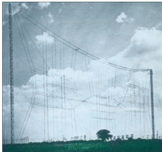
● Fig. 2: The Daventry transmitting 'beam' antennas circa 1937 - taken from a contemporary postcard (see text). Although no known photographs of the early antenna arrays at Wooferton were available to G3XFD - this array is fairly typical for the period.
