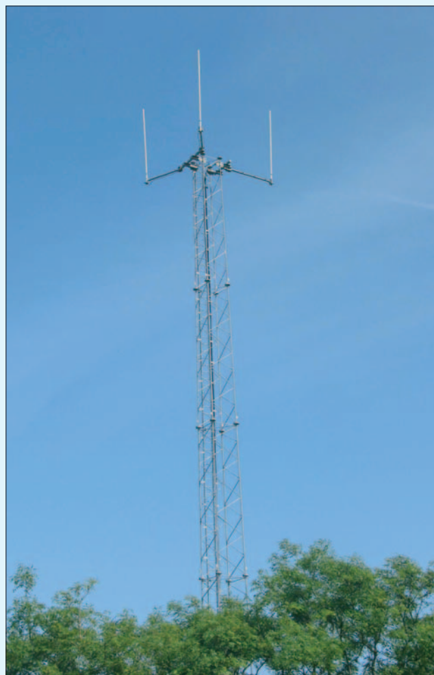
Fig. 1: This TETRA antenna was recently erected about 1 kilometre from Gordon's home in Brixham. With an operating wavelength around 0.75 metre and a gain of 8.5dBd (about seven times arithmetic ratio) the capture area approximates to 0.5 square metre.
