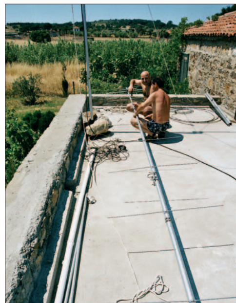
● The long boom of the 144MHz Yagi on the roof.
