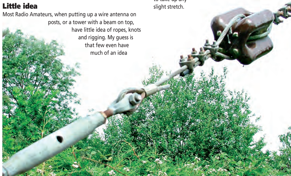
● Fig. 1: A close-up shot of the bottom end of a wire support rope where it attaches via the turnbuckle to a ground anchor. Note the three clamps on the two loops passing through the insulator. The commercial clamp is put on with such pressure as to form cold-weld junctions of the sleeve and rope for security.
