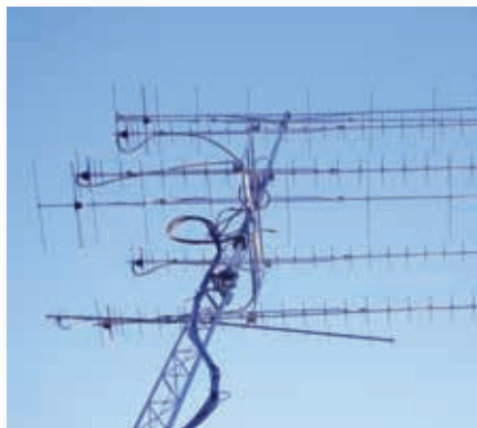
Fig. 1: The antenna system at the QTH of Reg Woolley G8VHI.
