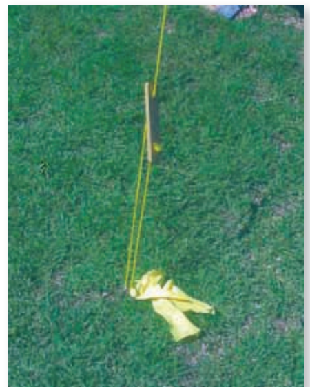
Fig. 3: Yellow flag markers show where the guy pegs are placed. The flags act as a warning to passers-by and also reduce the chance of the pegs being left behind.
