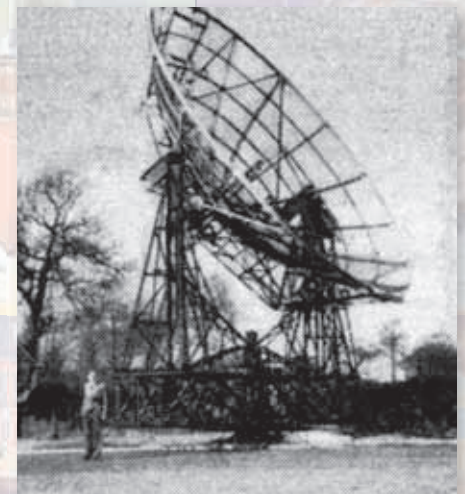
A completely steerable 30ft. parabolic reflector used as a radio telescope at the Jodrell Bank experimental station.
