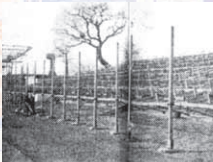
A partly adjustable broadside array of several hundred half-wave aerials.
