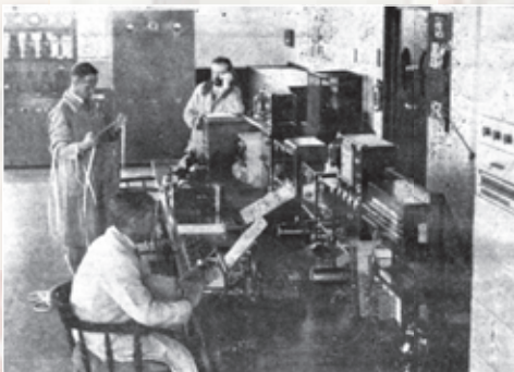
The control table for the transmitters of the new Police Radio Station at West Wickham, Kent.
