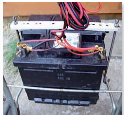
Fig. 8: A close look at the battery and the supply leads.
