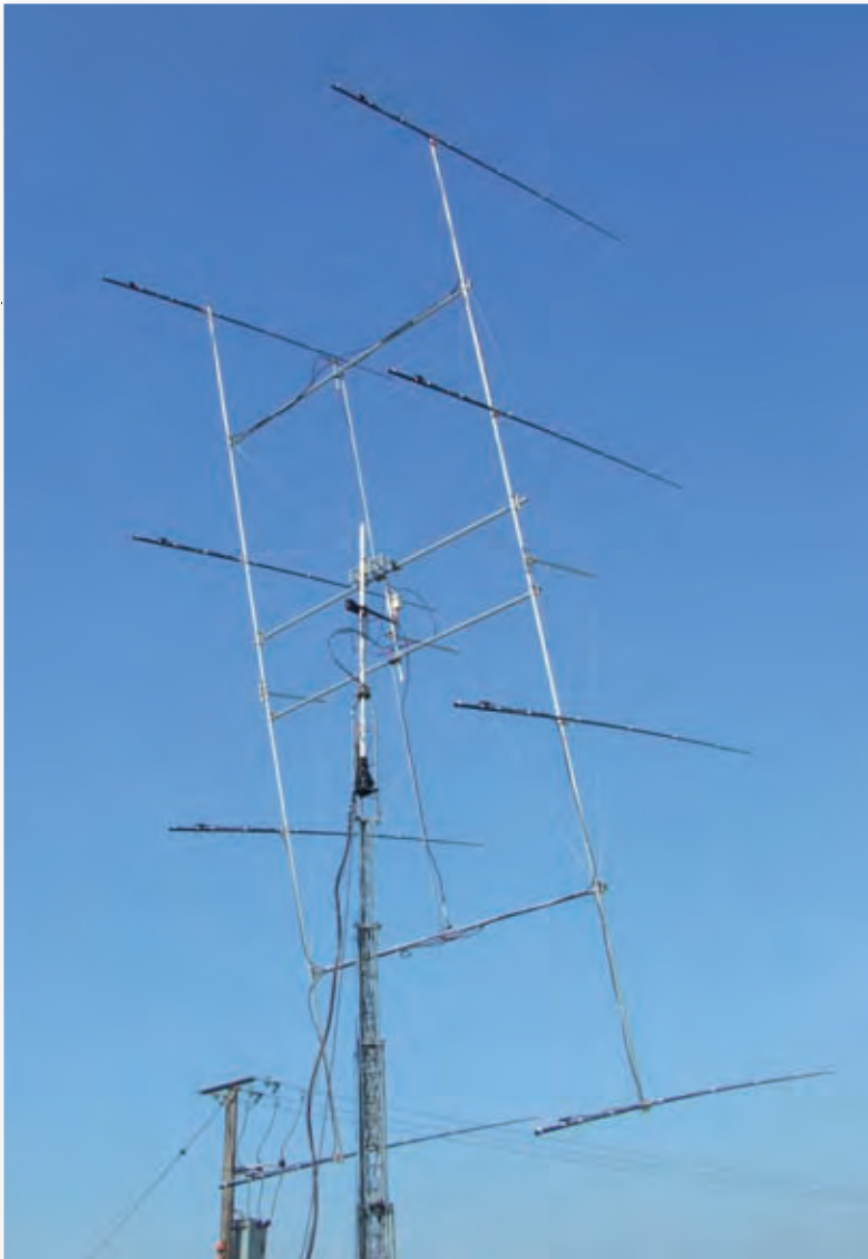
Fig. 1: The 144MHz antenna array at the QTH of David Johnson G4DHF
