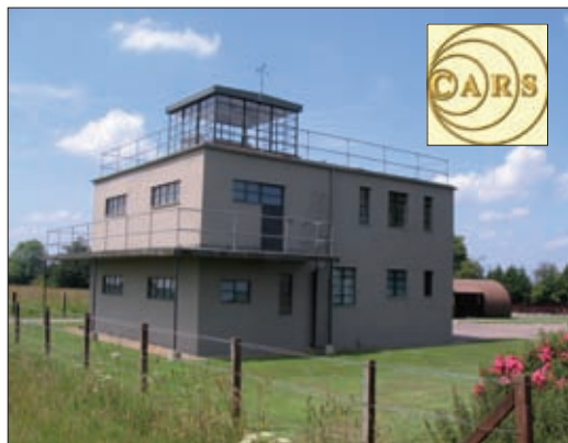
Thorpe Abbots Control Tower.
