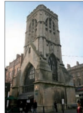
St. Michael's Church tower before restoration.
