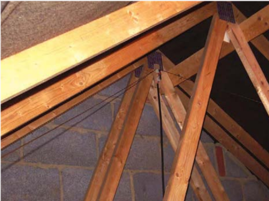
Fig. 7: Looking up into the apex of the roof, showing the inverted-V formed with the wires. The angle formed will most likely be different in house of different ages, as roof apex-angles have changed.
