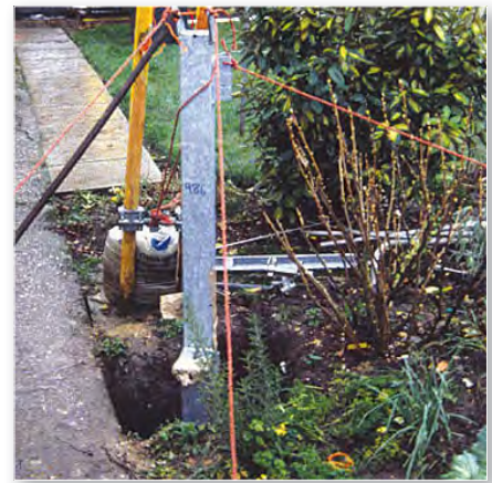
Fig. 6: To keep the mast vertical while the concrete sets, Colin G6MXL tied string around the post in the form of guys to temporary stakes in the ground.
