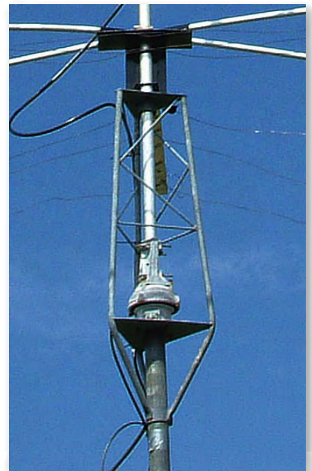
Fig. 2: Rotator Cage with the rotator mounted on the flat surface at the bottom of the cage, and the top of the cage acting as a support bearing.
