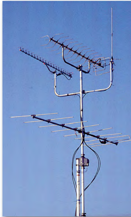
Fig. 3: The antennas are all pointing the same direction. In this installation the support bearing has been mounted below the rotator as the rotator has the antenna (stub) mast passing through it.
