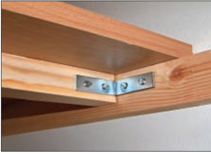
Fig. 2: An extra wooden bar added under the shelves for added support.
