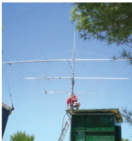
Spiros SV8CS finalising the installation of his 50MHz 7-element WOS LFA Yagi at his eco-friendly station.
