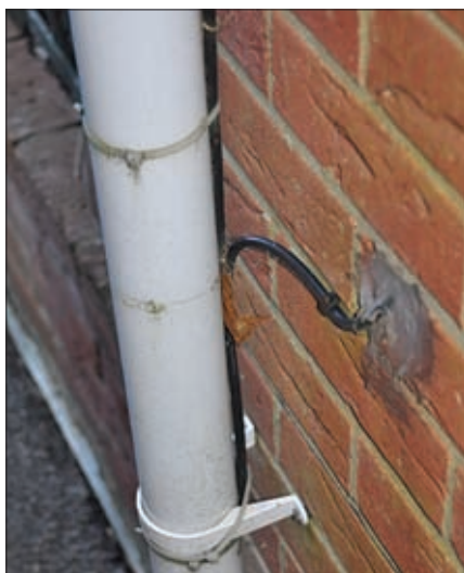
Fig. 6a: Feeder partially concealed behind a plastic downpipe. The black feeder used here illustrates the idea.
