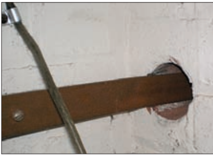
Fig. 1: A mousehole for the tape entry and exit. (The photos provide a clue to the nickname!).
