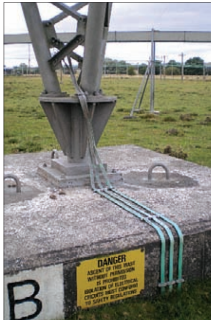
Fig. 3: When the output r.f. is contained within coaxial cables, provision is made to bond the mast itself to earth, here showing three such bonds.
