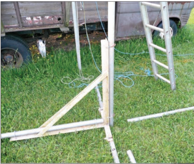
Fig. 3: The practical Gin Pole is now grounded after raising the mast to vertical. The pole running out of the picture towards you, forms a stabilising pivoting point, keeping the mast from falling sideways.
