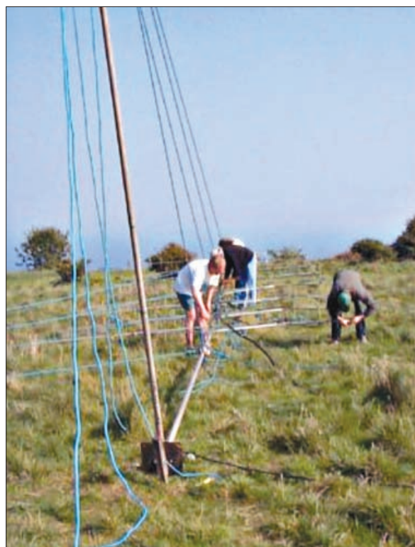
Fig. 2: Another view of the basic technique when using a Gin-pole.
