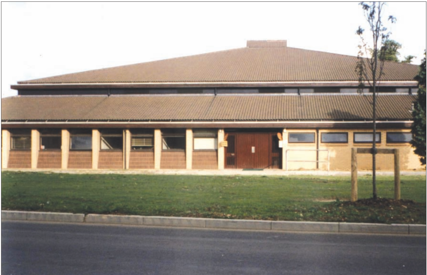
After the old CRS had been flattened, this was the new CRS building, which was opened on July 4th 1986. But only seven years later it had closed.
