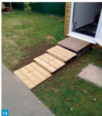
Fig. 6: Rafters in place. Fig. 7: With the roof in place. Fig. 8: The end wall half finished. Fig. 9: The ceiling timbers screwed into place (and resistor colour-coded!). Fig. 10: Carpeted and bench tops in place. Fig. 11: An idea of the internal decor. Fig. 12: Cable entry, seen above the trunking. Fig. 13: Steps for access. Fig. 14: The finished product.
