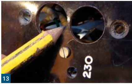
Fig. 13: This bridge to be removed.
